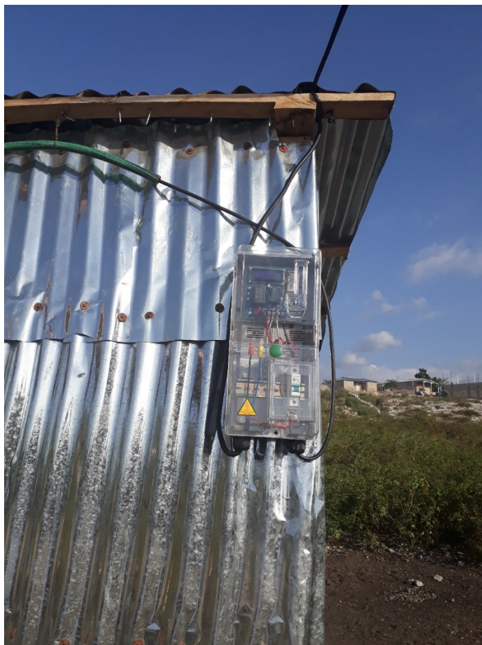
Image of a smart prepaid meter in operation in a small business in Mole St Nicolas. (Case of the SIGORA Micro-network, North-West, Haiti)
